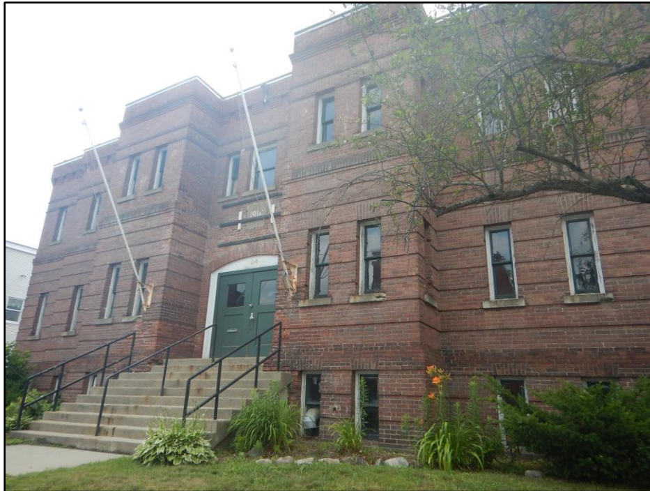
Photo 4. Photo shows the east side of the Armory building, facing Main Street. View is to the southwest.
