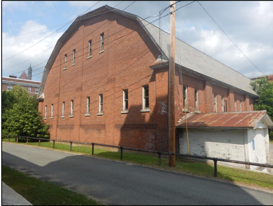
Photo 2. Photo shows the west side of the Armory building. View is to the northeast.
