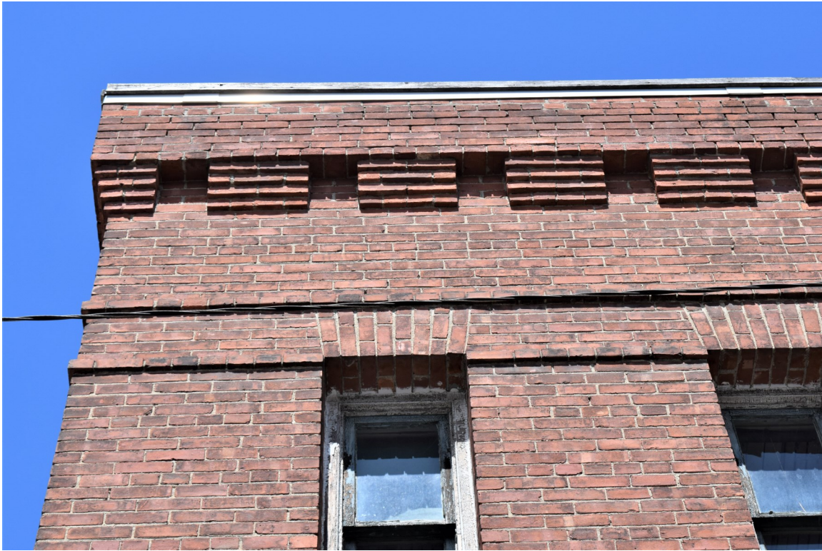
Photo 31: Looking west, view shows corbeled brick brackets under projecting bricked fascia forming the front block cornice
