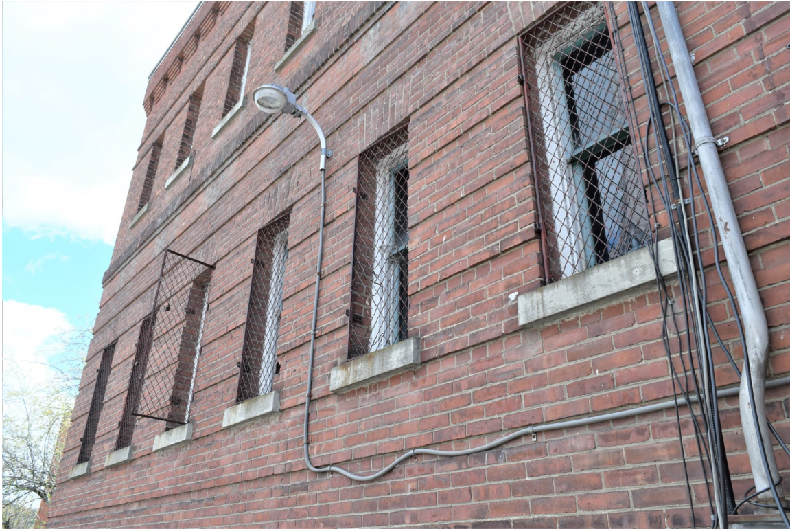
Photo 39: Looking southeast, view shows main block north elevation first floor sash protected by metal security grates
