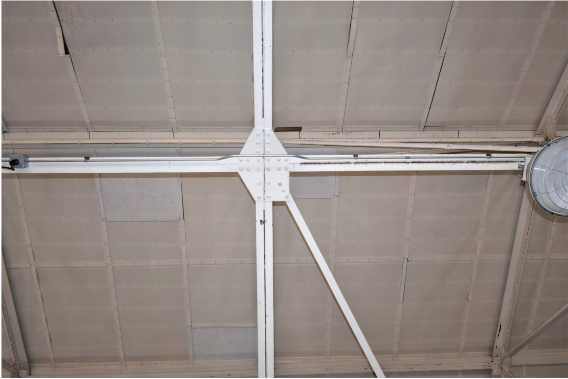
Photo 11: View shows drill hall roof truss and roof paneling detail
