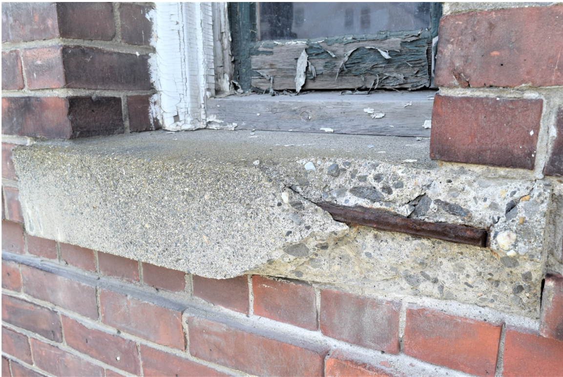
Photo 38: View shows main block window with deteriorated lintel and water related decay on lower sash
