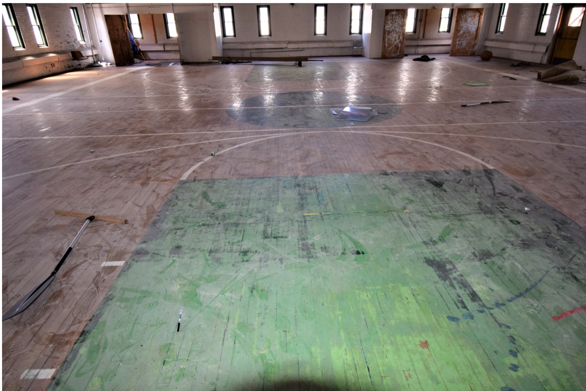
Photo 08: Looking west, view shows drill hall hardwood strip floor
