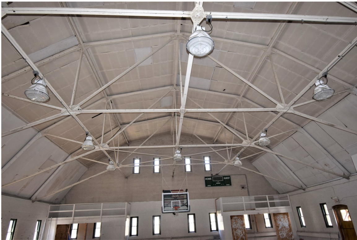
Photo 09: Looking west in drill hall, view shows built-up metal trusses supporting the slate-covered gambrel roof
