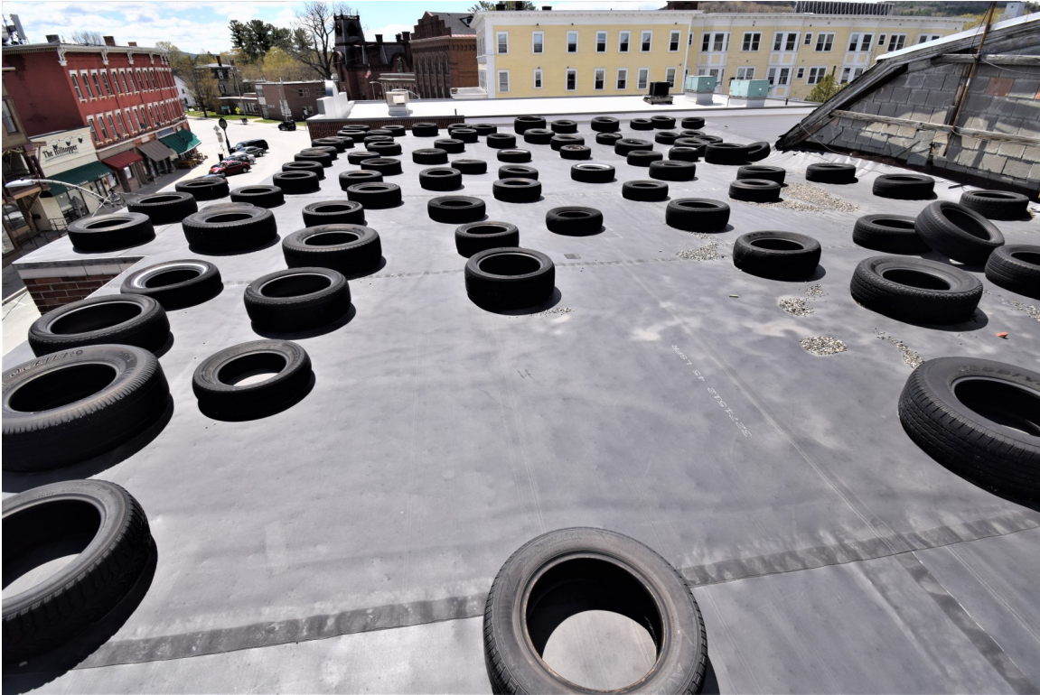
Photo 41: Looking south, view shows main block roof with temporary rubber membrane secured with rubber tires
