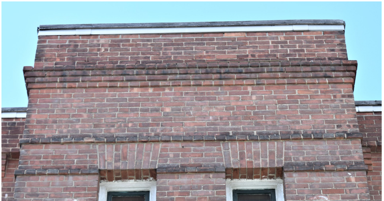
Photo 30: Looking west, view shows facade jackarch detail and decorative brickwork at roofline
