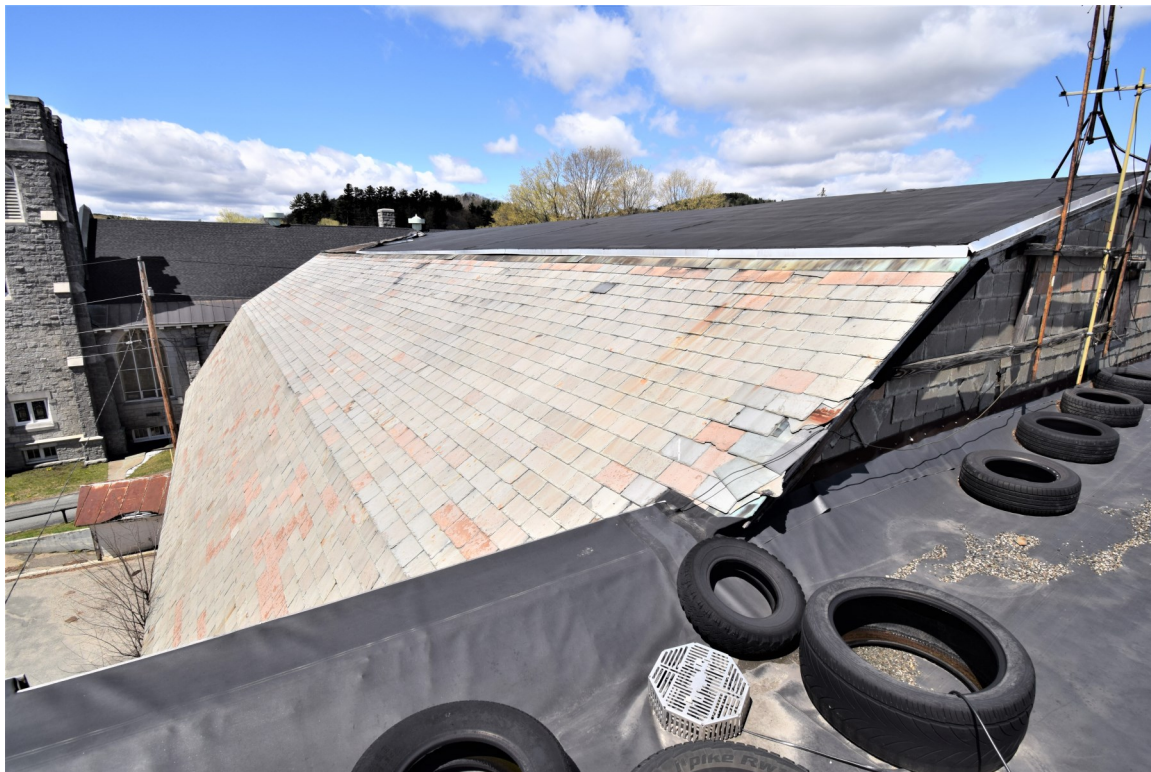
Photo 44: Looking west, view shows south side of rear block gambrel roof with the upper gambrel roof plane protected by a rubber membrane
