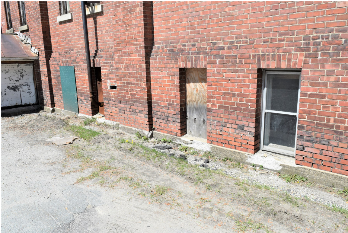
Photo 40: Looking northwest, view shows altered sash at rear block basement level
