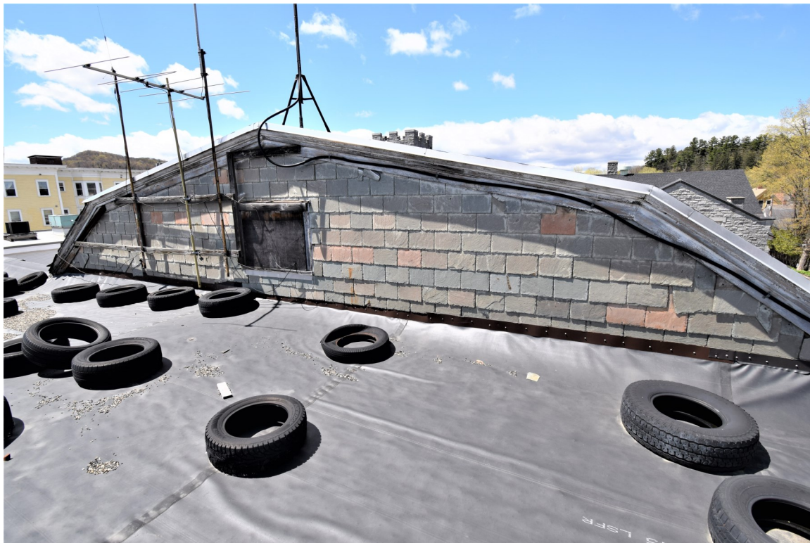
Photo 43: Looking southwest, view shows east facing exposed section of gambrel roof sided with slate
