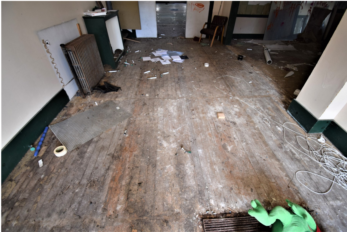
Photo 05: Looking west in room 1-1, view shows extant hardwood strip floor
