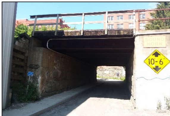
Figure 8: Honking Tunnel, July 2022
