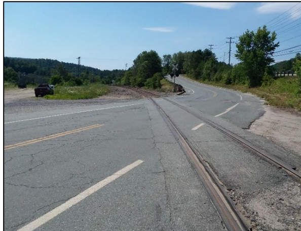
Figure 11: Rail Crossing at Bay Street
